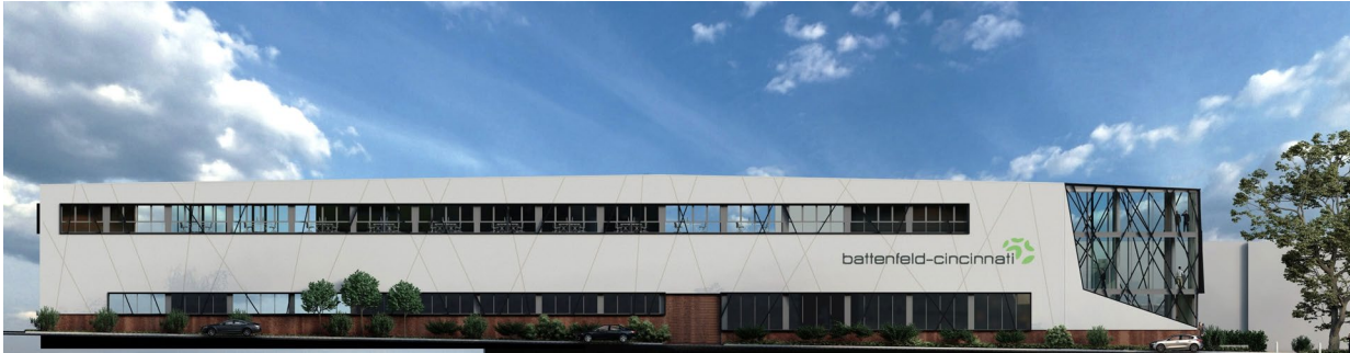
Technical center frontal view east side
